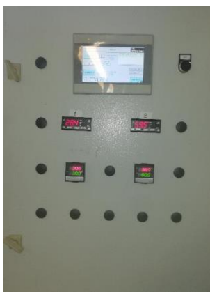
Figure 17. Pictures of the PLC and the central switchboard of the pilot plant
